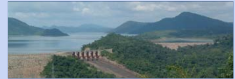
Figure 2: Multipurpose small and medium sized reservoirs in the upstream regions of the Volta Basin (first picture) directly competes with hydropower generation at the Akosombo dam (second picture) and smaller hydropower plants in the lower parts of the Volta Basin.
